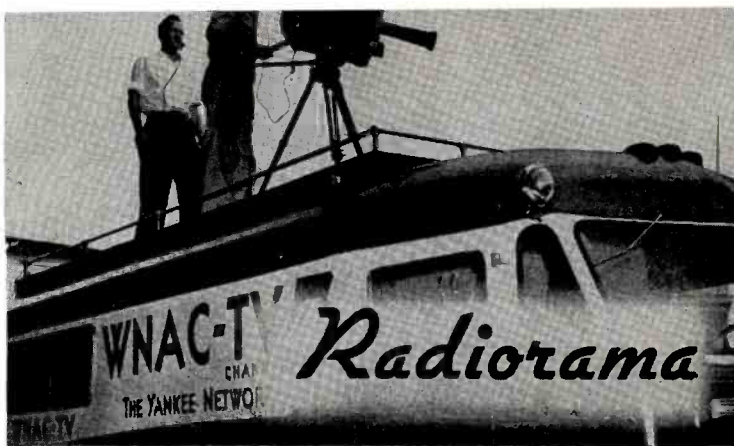
GENERAL ELECTRIC's new mobile television truck is put to good use by WNAC-TV Boston, the first to use the new unit. The truck's floor is 16 inches above the ground to facilitate loading and unloading of equipment.
